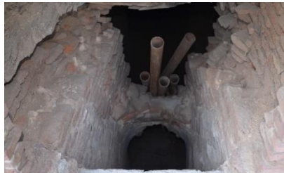
Figure 5 Basement chamber through courtyard (Source:Author)
